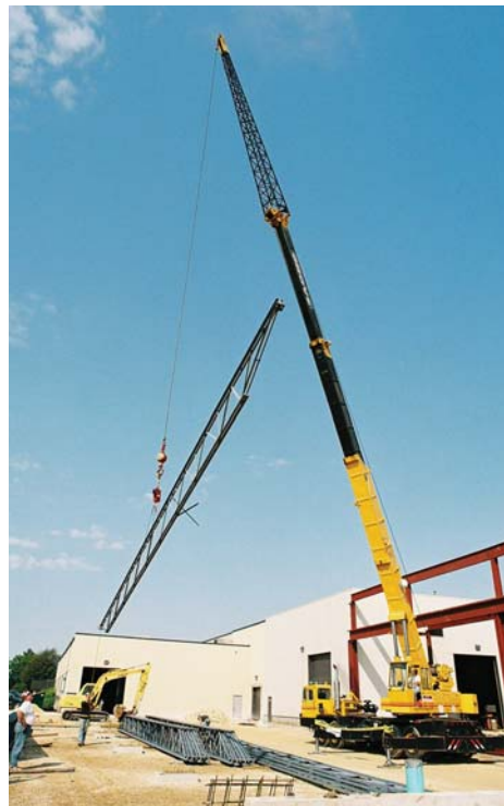
Setting trusses is a breeze
