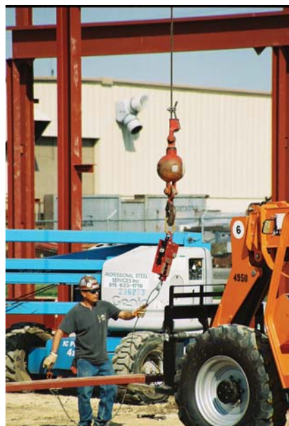
Setting header steel
