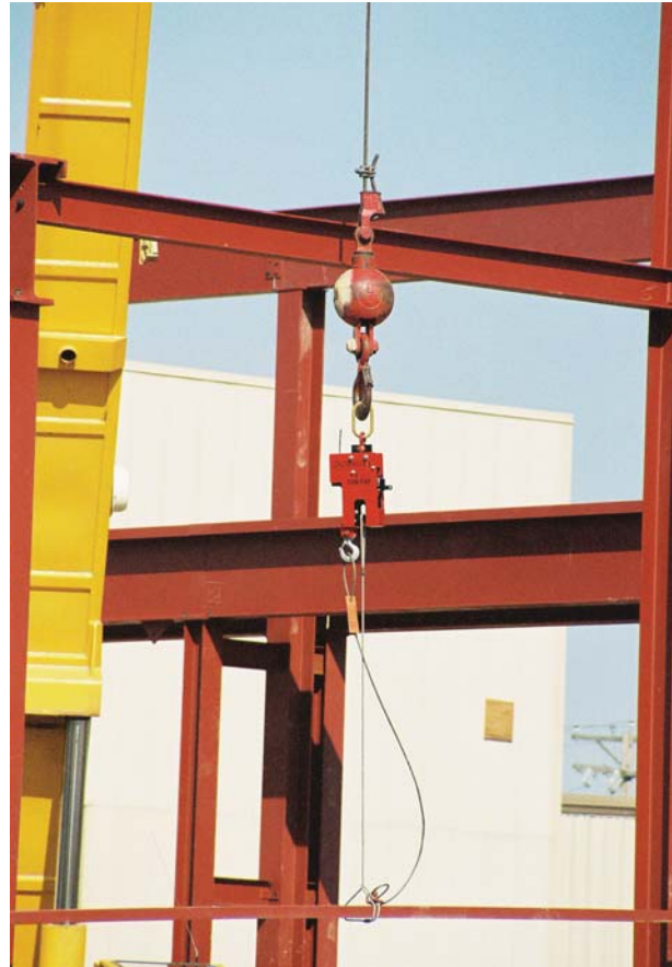
2.5 ton unit using a choker hitch
